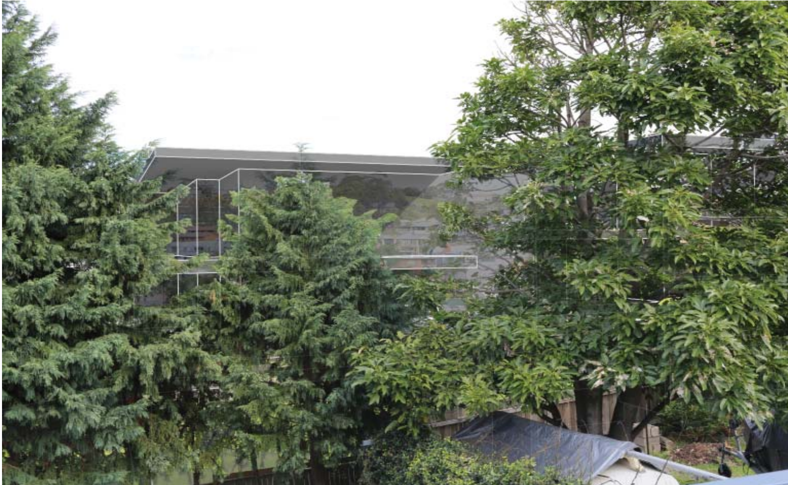
View from a rear upper deck of No.30 Minnamurra Street
